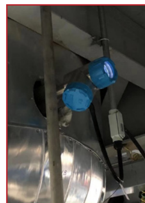
6.5 Reactor Side Installation
