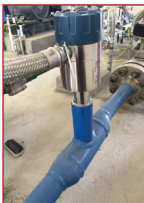
6.2 Threaded Installation
