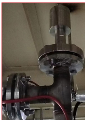
6.3 Elbow Pipe Flange Installation
