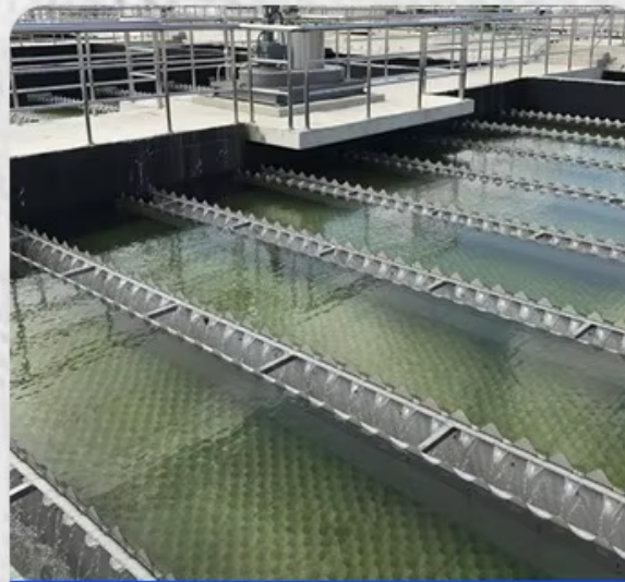
Sewage treatment plant
